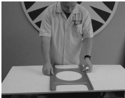
TB8 Tile Support Bracket used as a template
